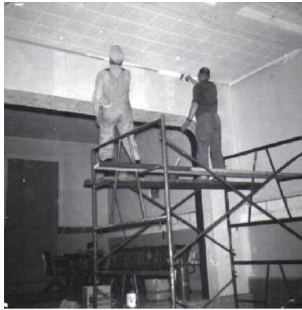
Preparing the old post office theatre
